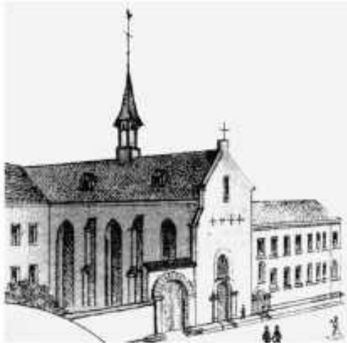
Chapel and abbey of the Alexian Brothers on the eastern side of Brückstrasse (now the Romaneum) around 1877
